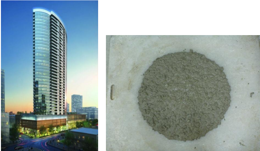
Figure 4. View of LPM Apartment Tower (photo credit of urbanmsp.com) and typical slump flow of developed HP-GSC
