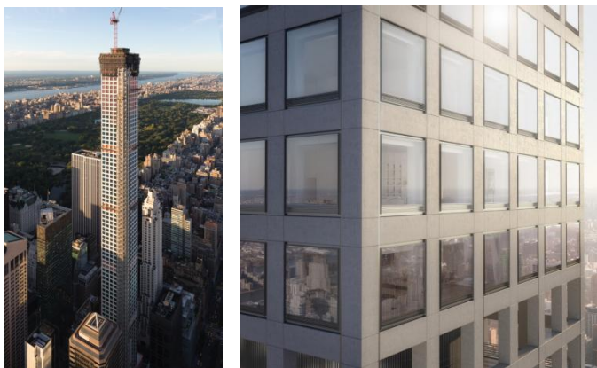
Figure 4. View of 432 Park Avenue apartment building and formed-surface finish cast with SCC (photo credit of Joe Nasvik [6])
