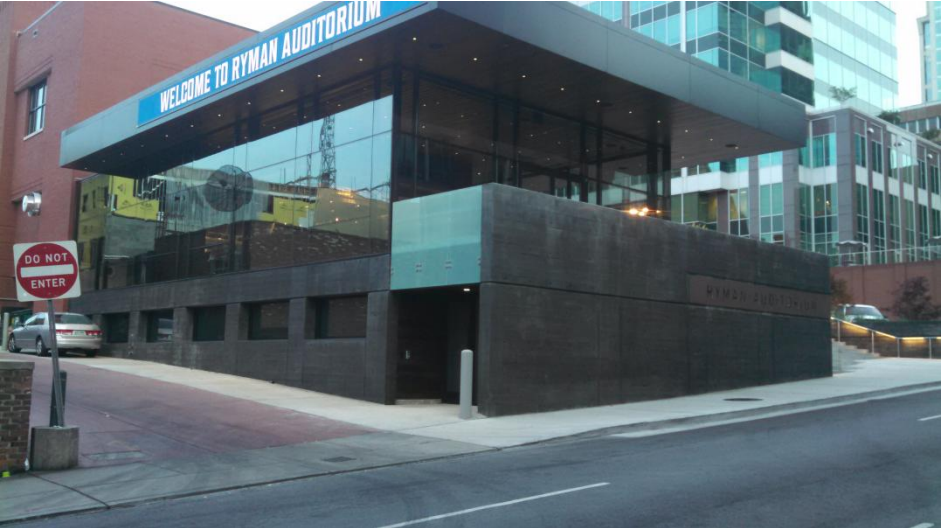
Figure 4. The completed Ryman Auditorium addition.
