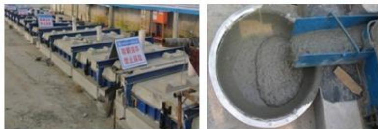
Figure 5. Full-scale experiment of SSFSCC construction
