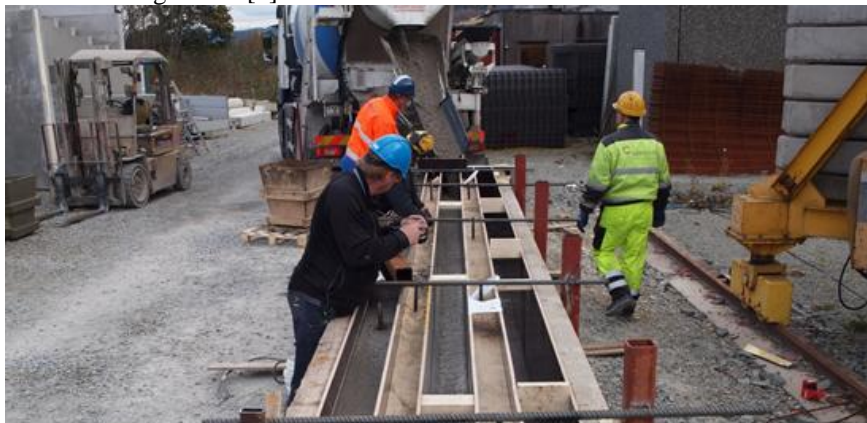
Figure 4. Casting of wall elements from truck gutter
