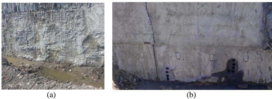
Figure 3. Full scale diaphragm walls cast with (a) Mix 1 (b) Mix 2.
