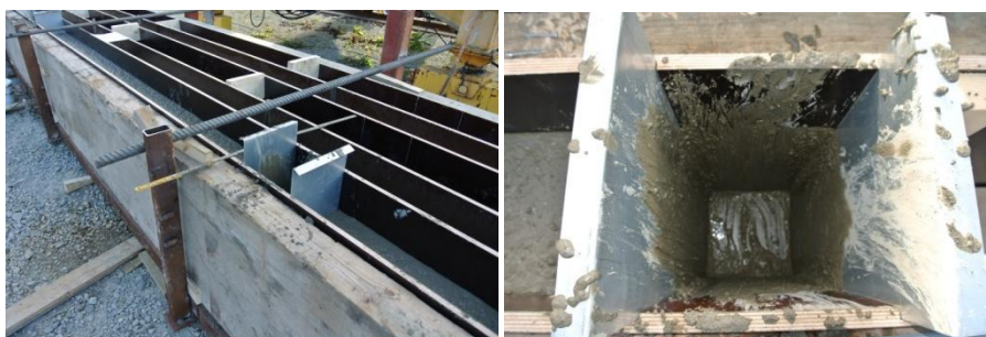
Figure 3. The wall elements with metal plates bounding the area for sampling
