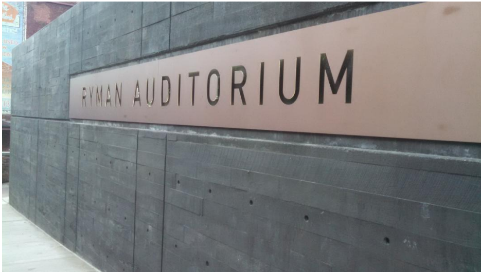
Figure 1. One of the completed rough-cut lumber formed walls with sign.
