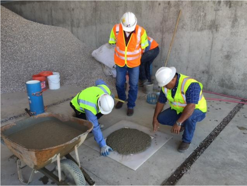
Figure 4. Slump-Flow testing as observed by DOT representative
