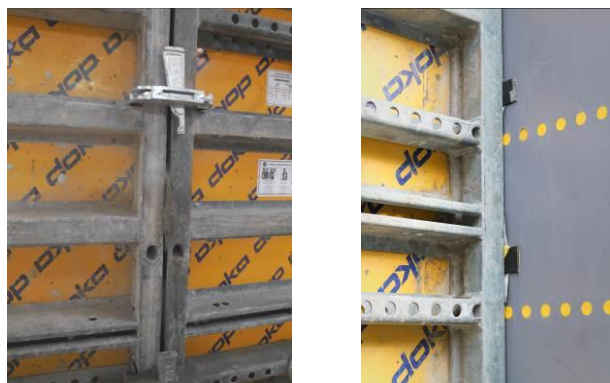
Figure 3. Butt joint (left) – Butt corner joint (right)
