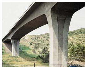
Sustainable HPC infrastructure
